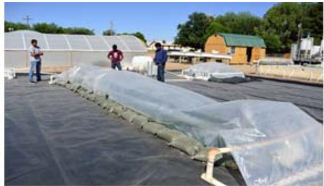
Figure 3. Fabrication of the enclosed photobioreactor for cultivating *Galdieria sulphuraria* in the POWER process.
