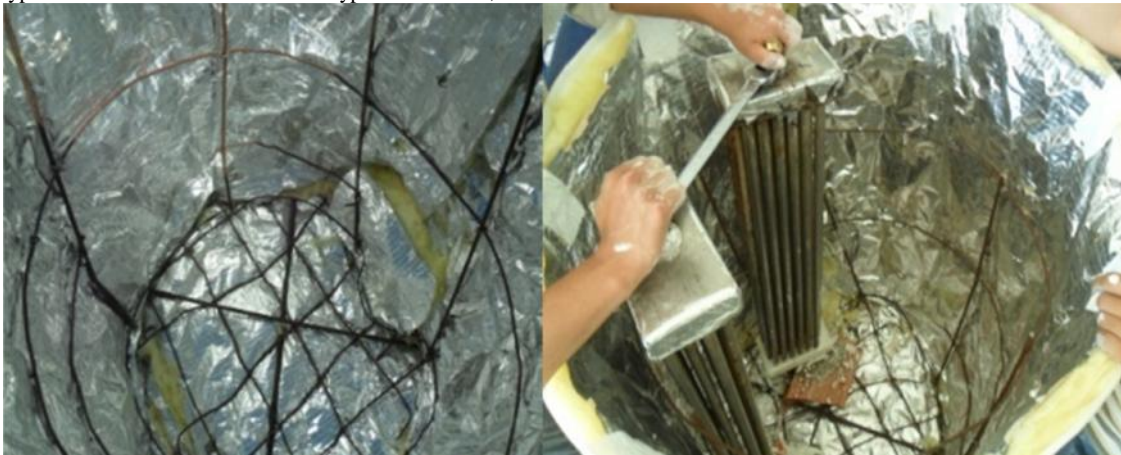
Figure 3: Preparation of the heat storage module
