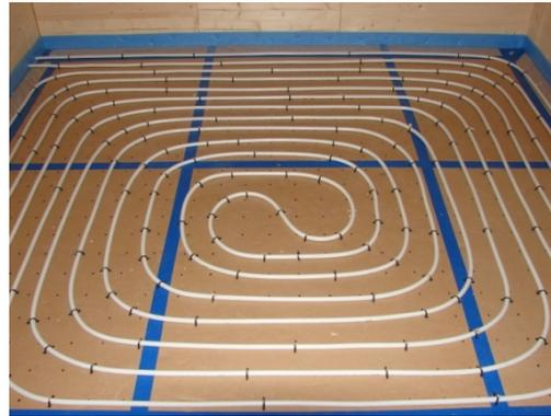
Fig. 7. The floor heating circuit
