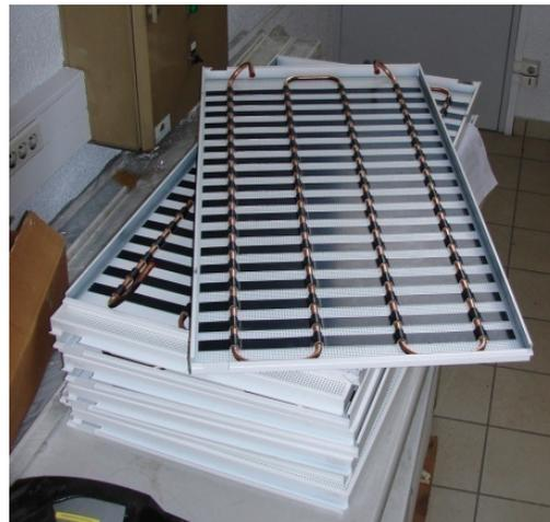
Fig. 8. The chilled ceiling plates
