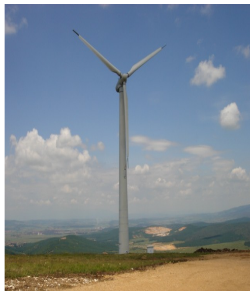
Figure 2: View of the installed wind generator
