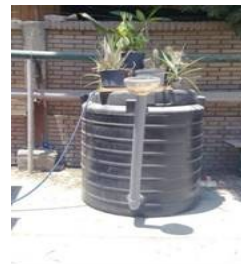
Fig. 20 Compact Bio gas unit
