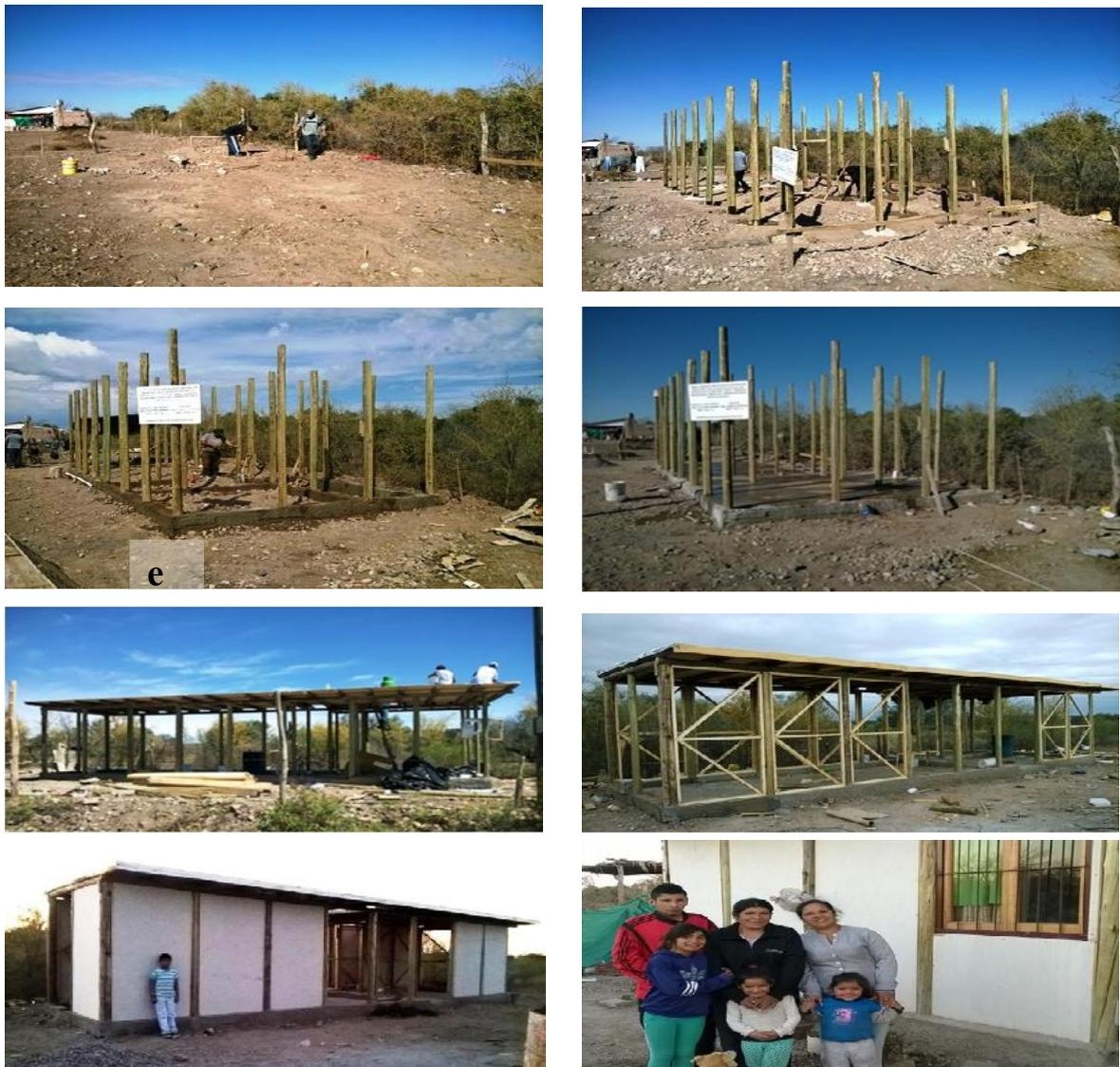
Figure 4: Housing Construction Steps
