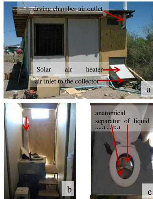
**Figure 7: Technology Used in Bath Room: A) North Façade of the House with Solar Collector of the Dry Solar Toilet System; (B) Toilet Seeing from Interior of Bathroom with Staircase of Access; (C) Anatomical Device to Separate Solids and Liquids**
