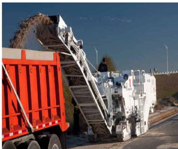
Figure 2 Milling of Asphalt Pavements (Courtesy of Roadtec)
